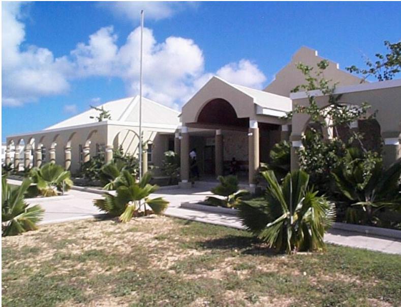
The New Anguilla High Court and Magistrate's Buildings
